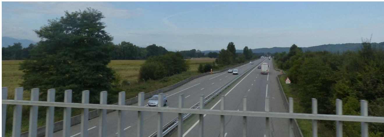
Illustration 21: Autoroute A64 (© Cabinet ECTARE)
