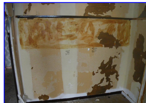
Joints de Placoplatre
